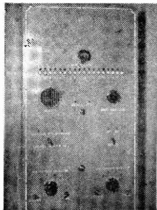
*The paging switch (centre left) carries out the complicated operation of cutting out all radio lines to speakers and paralleling them with the nurse's mike. It has 96 separate connections. The main panel is seen on the right.*
