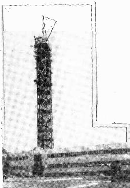
A 300-foot tower erected to house radio laboratories at Nutley, New Jersey. A total of 800 tons of steel was used for this tower, built by the U.S. Steel's American Bridge Company. Experiments carried out in this tower will probably make possible broadcasting of many programmes on a single channel, and multi-channel telephony by pulse time modulation.
