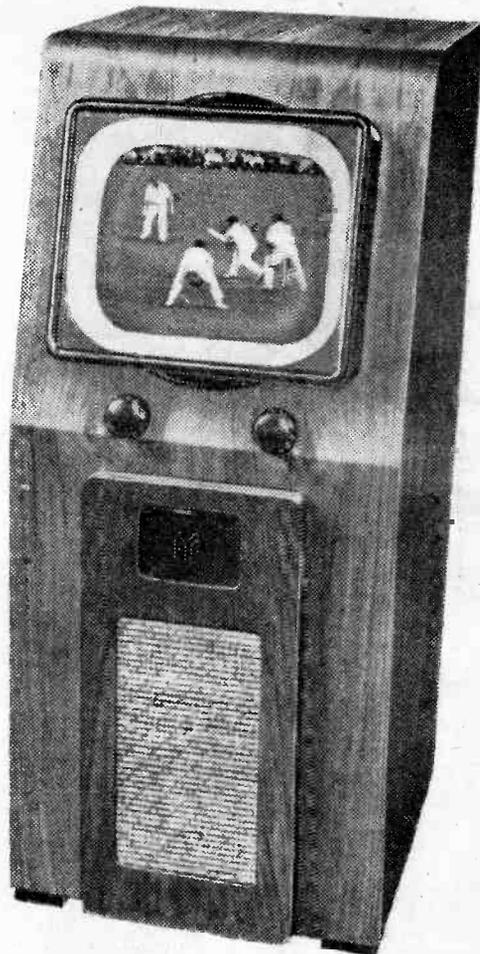
A Pye television receiver of the console type. Although having only two controls (Brightness and Volume) the remaining controls, such as Contrast, Line Hold, etc., are accessible, being mounted immediately behind the small panel seen below the two control knobs. Thus it is a simple matter to make adjustments as and when required. This model gives a black-and-white picture.
