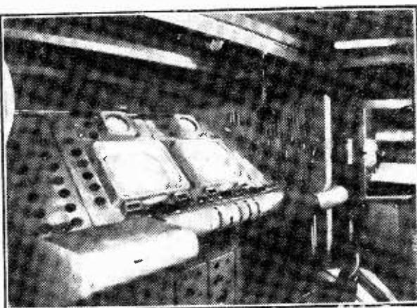
The interior of one of the new Pye Mobile Television units. This is housed in a "shooting brake" type of car with telescopic reflector type aerial mounted on the roof.
