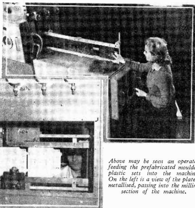
Above may be seen an operator feeding the prefabricated moulded plastic sets into the machine. On the left is a view of the plates, metallised, passing into the milling section of the machine.
