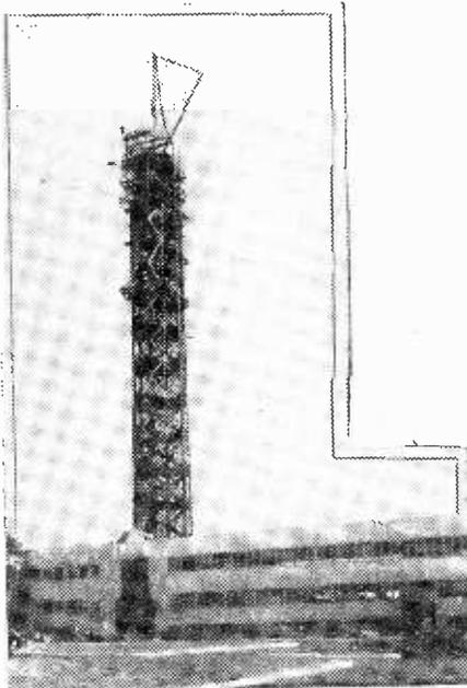
A 300-foot tower erected to house radio laboratories at Nutley, New Jersey. A total of 800 tons of steel was used for this tower, built by the U.S. Steel's American Bridge Company. Experiments carried out in this tower will probably make possible broadcasting of many programmes on a single channel, and multi-channel telephony by pulse time modulation.
