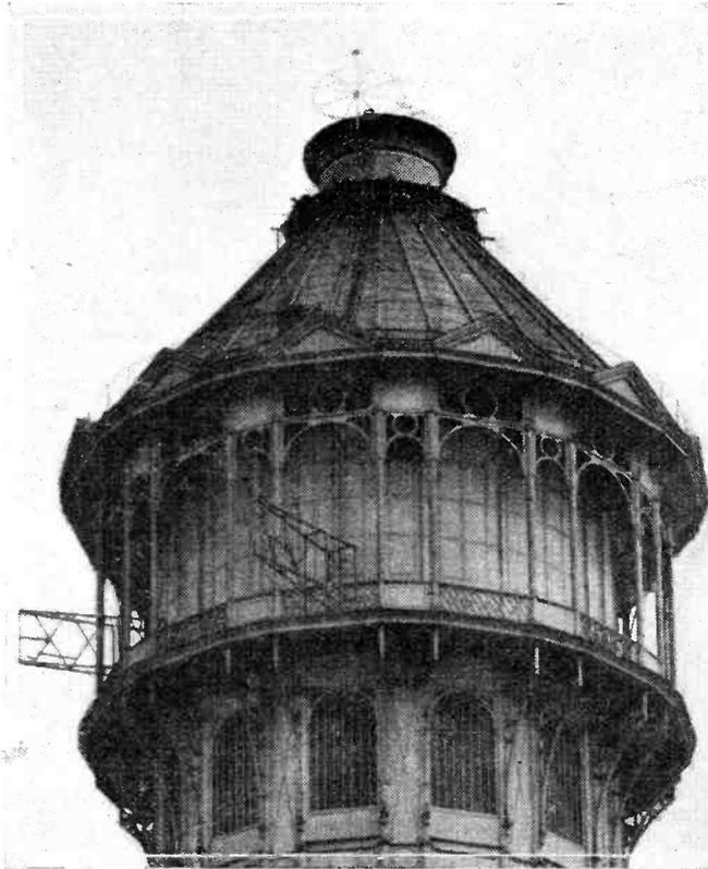
*A good example of a spoked aerial array capable of giving efficient radiation in a horizontal direction.*
