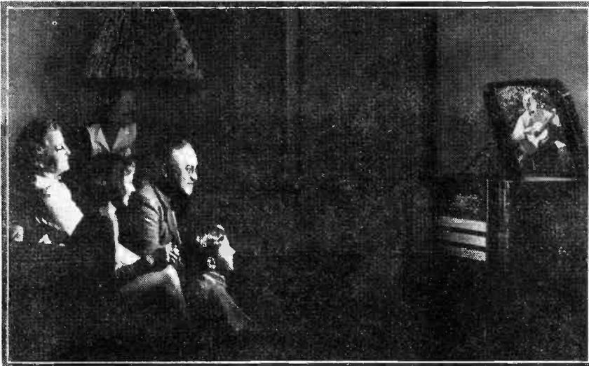
Fig. 2.—The compact projection type television receiver, with reflecting screen, in use in the home.
