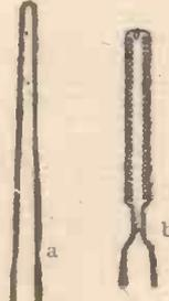
Fig. 5.—Straight and spirals types of heater.
