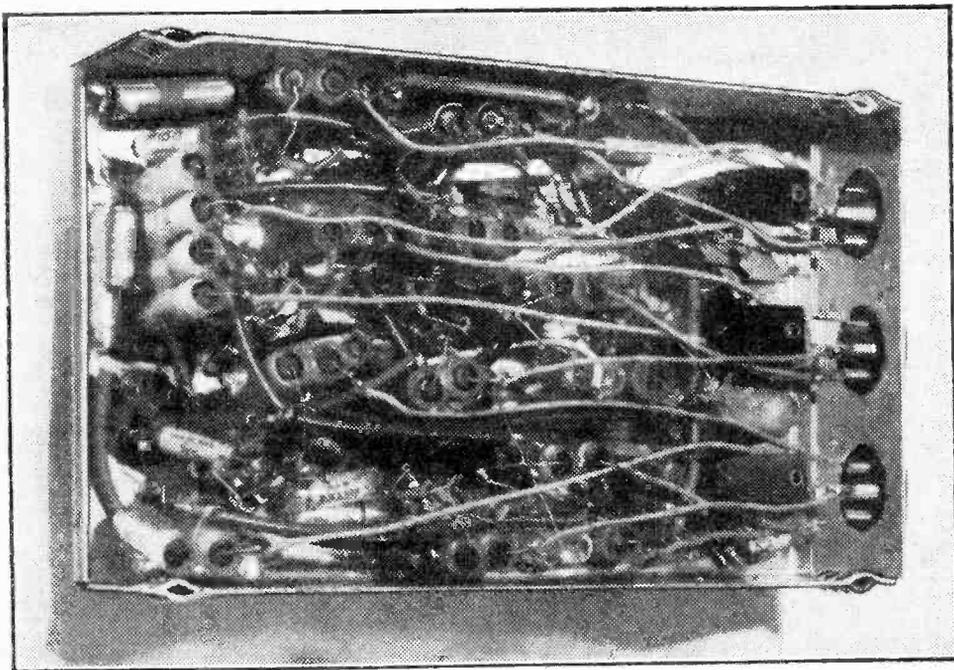
*This view of the underside of one of the chassis shows the condenser blocks and general layout.*
