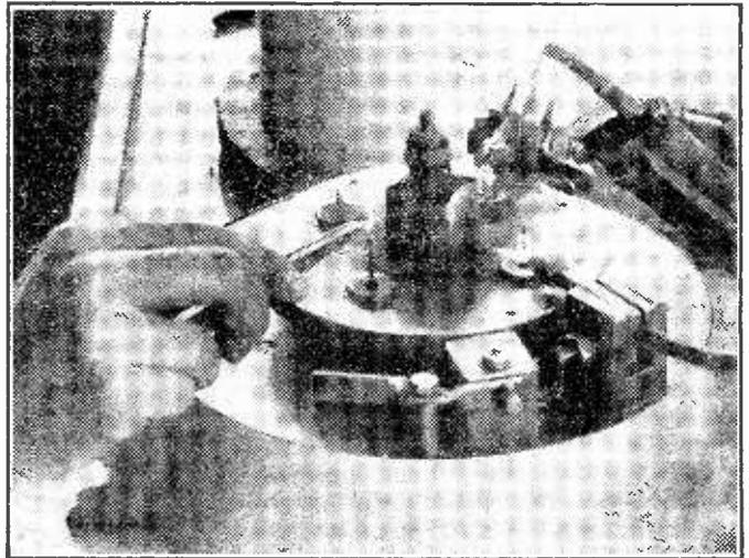
Fig. 1.—Fusing the glass capsule of the G.E.C. germanium diode to the alloy tube. An oxy-coal-gas flame is used and the machine is semi-automatic.
