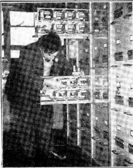
A technician replaces an output unit into the radio distribution unit of a channel used by controllers speaking to aircraft. (See "Air Traffic Control".)
