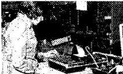
**Signs of things to come. A complete data terminal in an attache case. It comprises a full keyboard, all necessary electronics, and a small collapsible television screen which folds down. The station may be used over a standard telephone via a modem, and can chat to computers and data terminals anywhere in the world**
