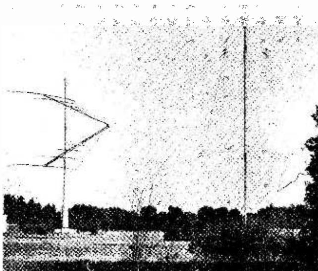
**Two aerials at the Austrian Radio Transmitting Centre in Moosbrunn, Lower Austria. On the left, a log-periodic for beaming signals to distant targets, on the right an omni-directional cage antenna for European broadcasts**
