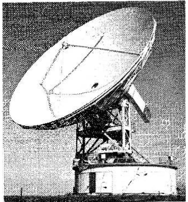
**Goonhilly 4 (11/14GHz) is currently proving digital satcom. technology with the OTS2 satellite**
