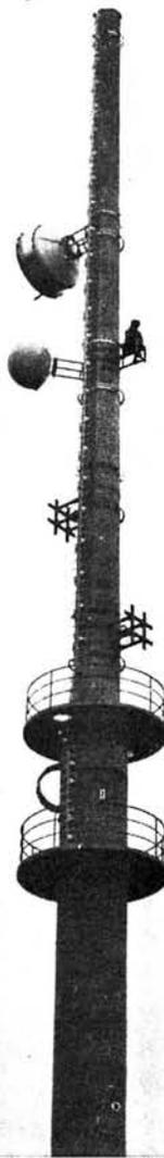
**A microwave antenna being mounted onto one of the modern concrete pylon towers preferred by environmentalists**
