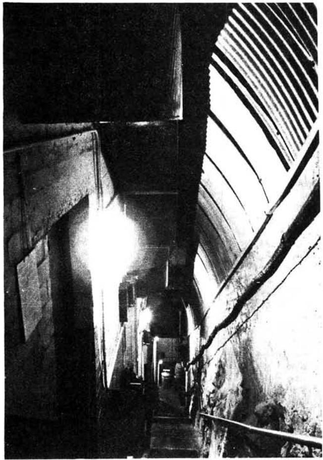
**The stairway looking down with the transmitter room door in the left foreground. Main extract ducting is overhead and note the living rock behind the handrails on the right. The corrugated iron sheeting on the above right is to prevent water dripping through into the tunnel**
