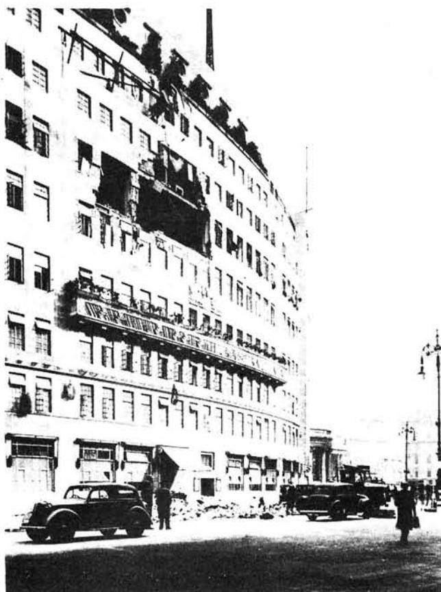
**London's Broadcasting House damaged by enemy action. A delayed action bomb came through the telephone switchboard room on the 7th floor and landed in the Music Library on the 5th floor at 2010. It exploded at 2102 and blew out through the News Department on the west side of the 5th floor. Listeners to the 9 o'clock news heard the announcer pause and then continue with his reading**
