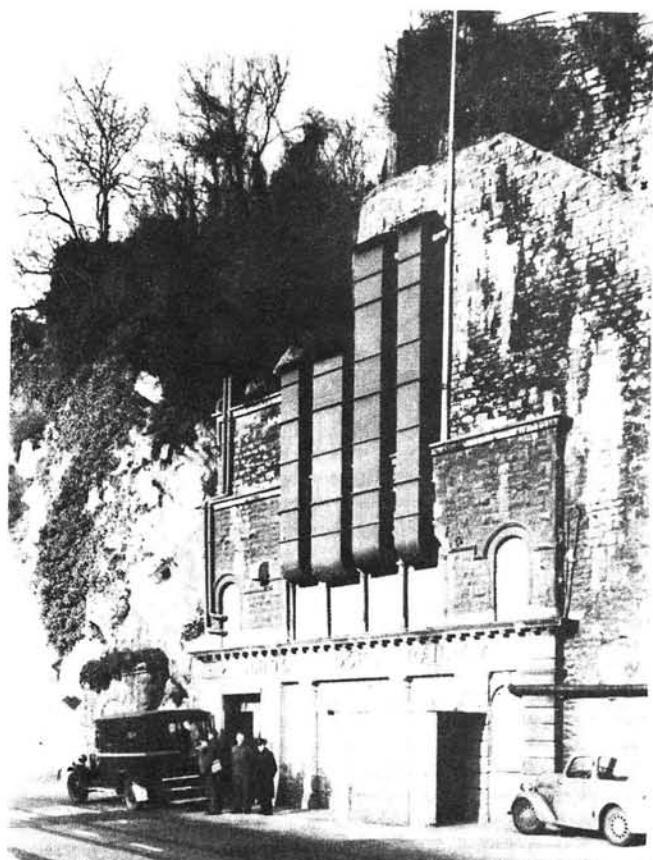
**The entrance to the BBC's wartime Bristol HQ showing ventilation intake and outlets. Adjoining these on the right is the antenna mast for reception**
