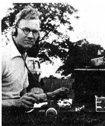
**Yours truly, G4AR, operating the Dollis Hill RC NFD station in June 1939. Note the Vibroplex bug key, dry battery (120V) for the transmitter and receiver and the mighty changeover switch! The accumulator for the 2V filament valves was on the ground. Fellow club member Fred Crane has just unearthed this and other NFD photos from his album after 45 years!**
