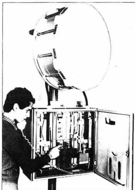
*GEC 19GHz narrowband digital microwave radio equipment*
