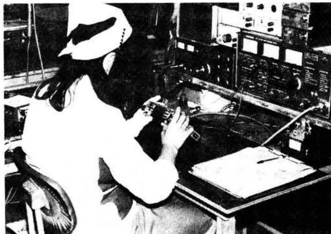
A Yaesu transceiver on final test
