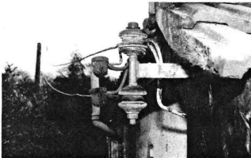
The PME system uses the supply neutral conductor to provide a low impedance pathway for fault currents.
