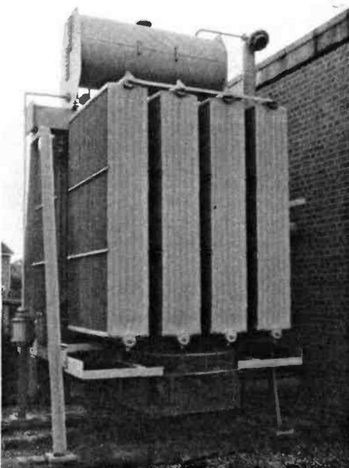
With the PME system, fault currents have a low impedance return path to the local transformer and protective switchgear.
