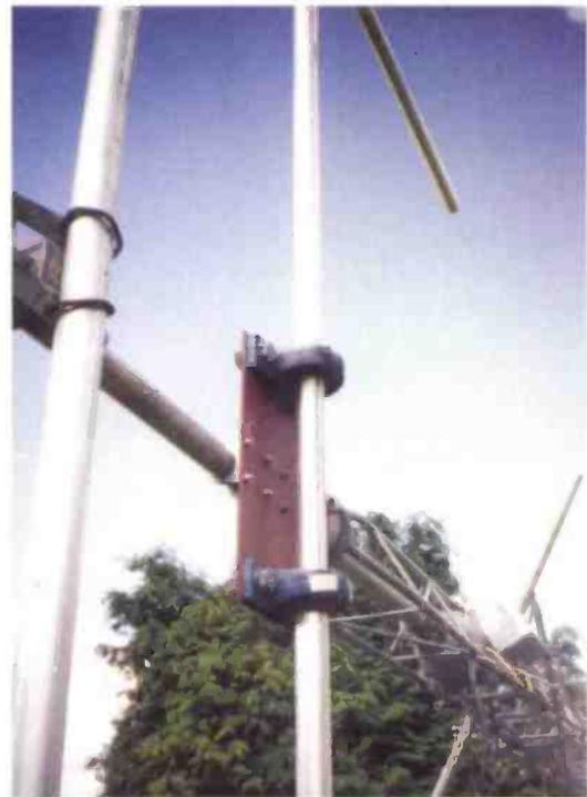
Fig. 4: A robust pivot bearing may be needed in some circumstances. See text for a slightly cheaper alternative that may be adequate for your needs.
