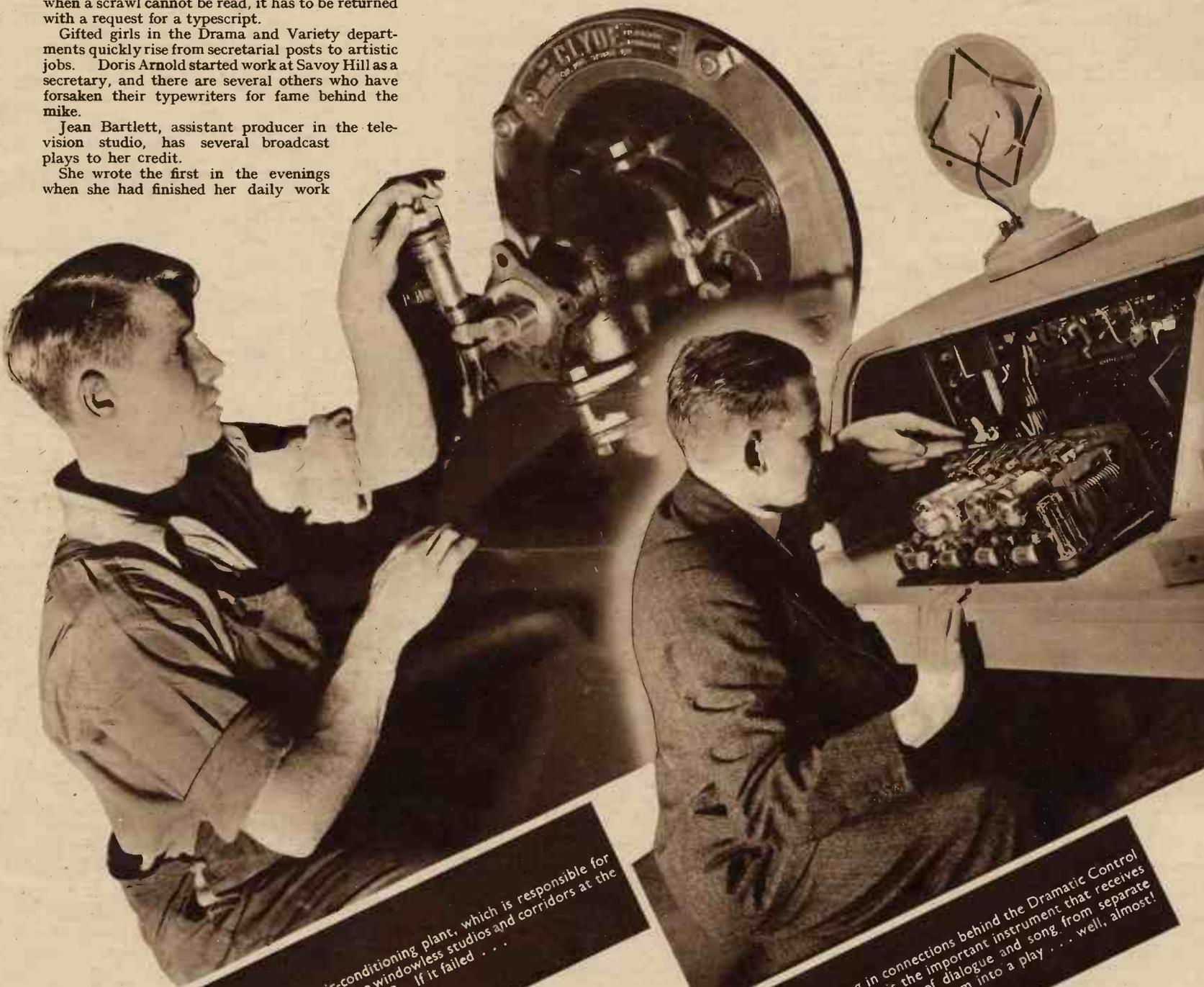
Greasing the air-conditioning plant, which is responsible for pumping air into the windowless studios and corridors at the B.B.C. If it failed . . .
