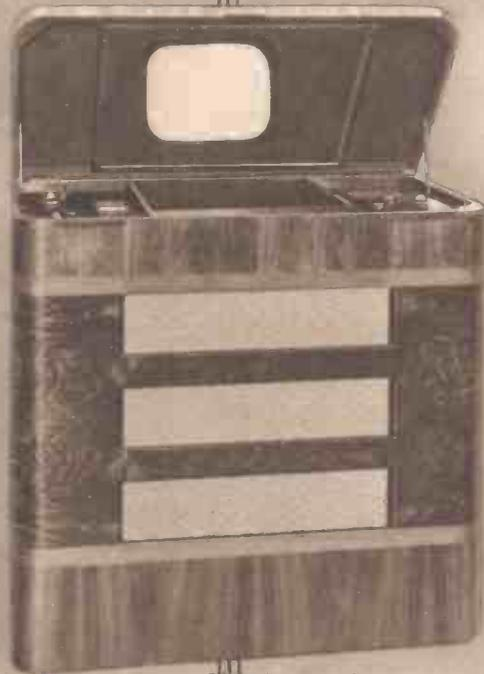
All major controls are mounted on instrument panels on either side of the vertically mounted tube. In this G.E.C. instrument the picture is viewed from a mirror mounted in the lid
