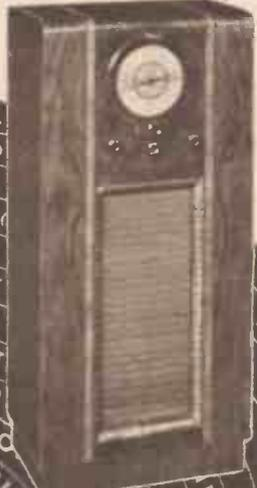
**PILOT B.344.** A Battery operated 4-Valve All-wave superhet with a performance comparable with main sets. The *Wireless World*, after testing this model said, "Not the least difficulty was experienced in obtaining reliable reception of American broadcast as well as of all the principal Continental short-wave stations."
