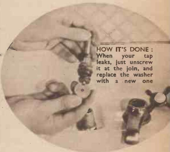
**HOW IT'S DONE:** When your cap leaks, just unscrew it at the joint, and replace the washer with a new one
