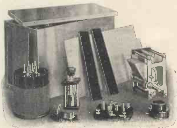
Before proceeding with the construction of the screened units the components for each should be collected together as shown in the above illustration.
