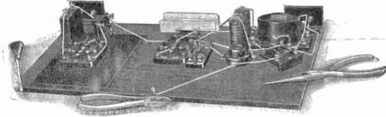
**S**HOWING the baseboard components placed into position and partly wired-up. Here the dual mounting of the specified valve-holder is to be seen. That for the screened-grid is vertical. It is mounted flat for the Mullard Pentone. The illustration below shows a closer view of the panel.
