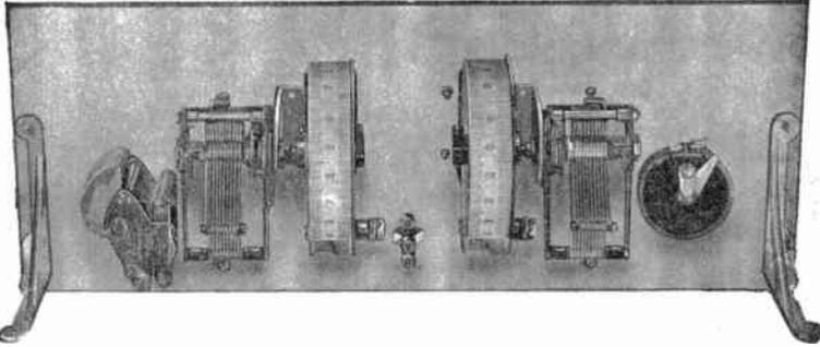
**FROM** this viewpoint, the longer contact leaf of the battery on-and-off switch would be on the right hand side of the switch spindle.
