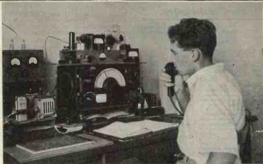
MD2C, Tripoli, has an R1155 receiver and runs 22 watts input to a two-stage transmitter. The operator is ex-G3BCY.
