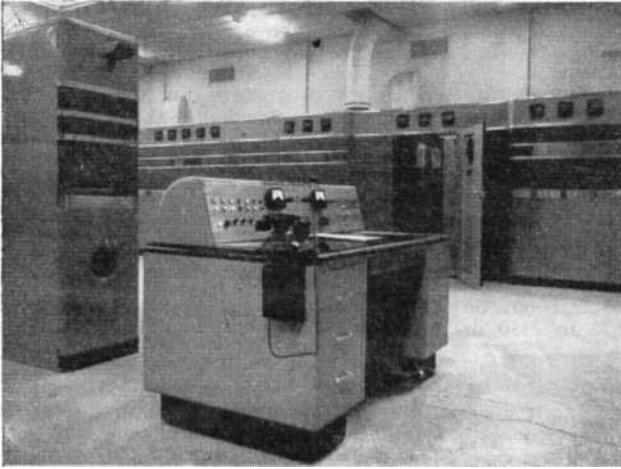
The 50-kW RCA transmitter for VLC, Radio Australia, with monitoring equipment and control desk in the foreground.
