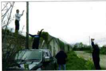
Some of G3SWM's motley crew doing a bit of antenna erecting for the listening contest on Portland.
