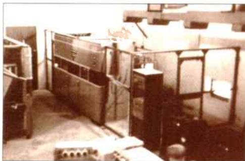
One of the three RCA 7.5kW transmitters.
