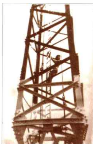
Starting to climb an antenna tower.
