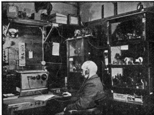
1.7, 3.5 and 14 Mc, on which he is normally active. The 14 Mc rig is the QRO job, CO-FD-BA-PA, with 100 watts input to the pair of '10s in the push-pull final amplifier.
