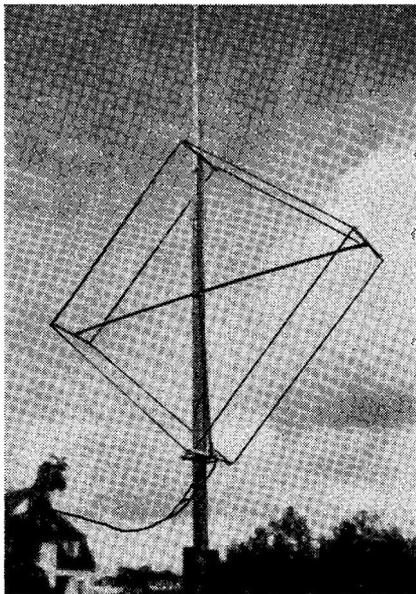
G2MV's square-beam aerial, lowered for inspection. The elements between the cross-pieces are  $\frac{1}{4}$ -wave for the frequency, and maximum directivity is broad-side to the array.
