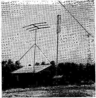
General view of G6CU/ZC2, the famous station on Cocos Is. The 3-element rotary is beside the hut, and the 105 ft. tower in the background carries the Sterba array, put up latterly.
