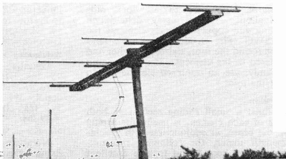
Close up of 4-element wide-spaced 58 mc beam at G5BY, carried on a 12 ft. mast during alignment tests.
