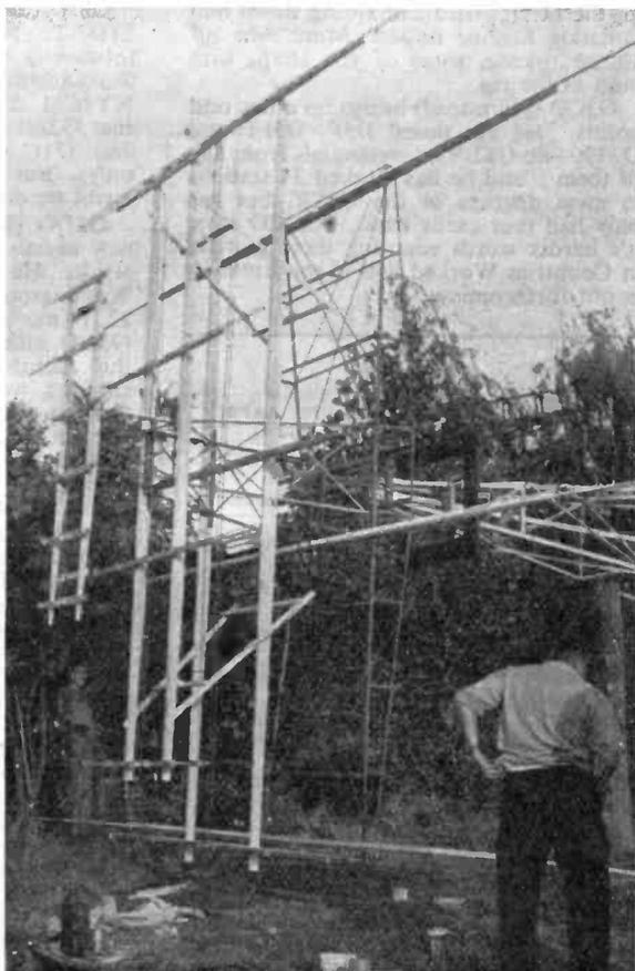
Not a disaster, nor yet a radar aerial array, but the top of VK3KU's composite rotary beam for 14, 28, 50 and 166 mc, lowered for inspection.
