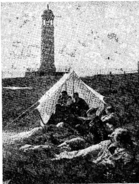
The lighthouse supports the far end of a 1.7 mc 1-wave aerial (264 ft.), and the operators on this station worked in shifts.
