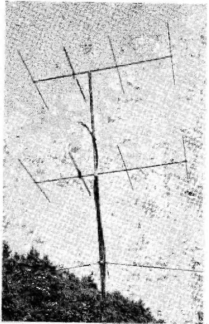
Dual 4-element wide-spaced beam stacked and fed in phase, G4CI, New Malden, Surrey. Radiators are arranged to present 100 ohms at their feed points, individually. The  $\frac{1}{2}$ -wave section joining them has a surge impedance of 155 ohms; this operates as two independent  $\frac{1}{4}$ -wave sections giving an impedance rise up to 200 ohms at the point where the feeder is connected.
