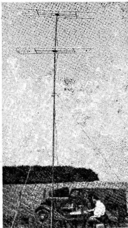
General impression of G5RP/P on July 3. The beam consists of two sets of two half-waves in phase.
