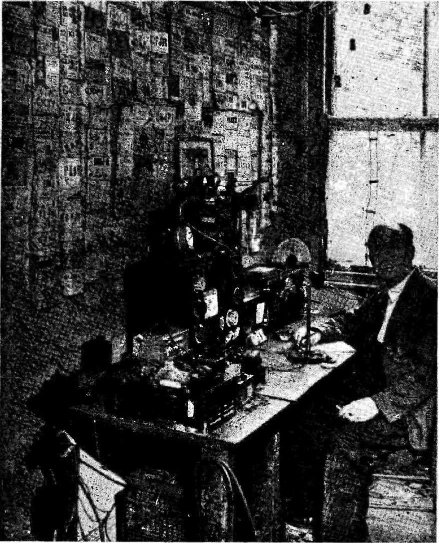
At G8IX, Hanley, Staffs. the transmitter is a T.1154 with an 1134A modulator, running 70 watts phone and 100 watts on CW; receiver is an 1155 modified with bandspread, and the main aerial a 132-ft. Windom. G8IX started his radio career in 1915 as a boy telegraphist in H.M.S. "Diana," and during the last war was a Sea Cadet instructor.
