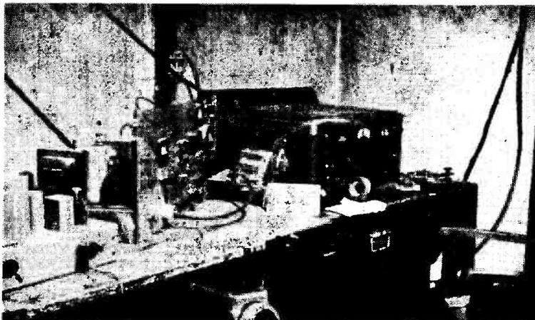
ZC1AZ as operated at Amman, Transjordan, for the two years to January, 1950. An 813 PA produced the RF on 14 and 28 mc, CW and Phone, with a pair of 805's in the modulator. Receiver was an SX-28, aeriels various (including a beam for Ten), and the operator of ZC1AZ is now G3GTA (Bath).
