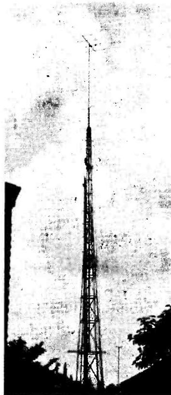
The G5YV beam head at the 62-foot level—still with 30 odd feet in hand to wind up. In other words, the beam can be pushed up half as far again! The "thickness" up the mast (which actually tapers gracefully and is a first-class engineering job) is a 42-ft. pole in the background which happens to coincide with the camera angle.
