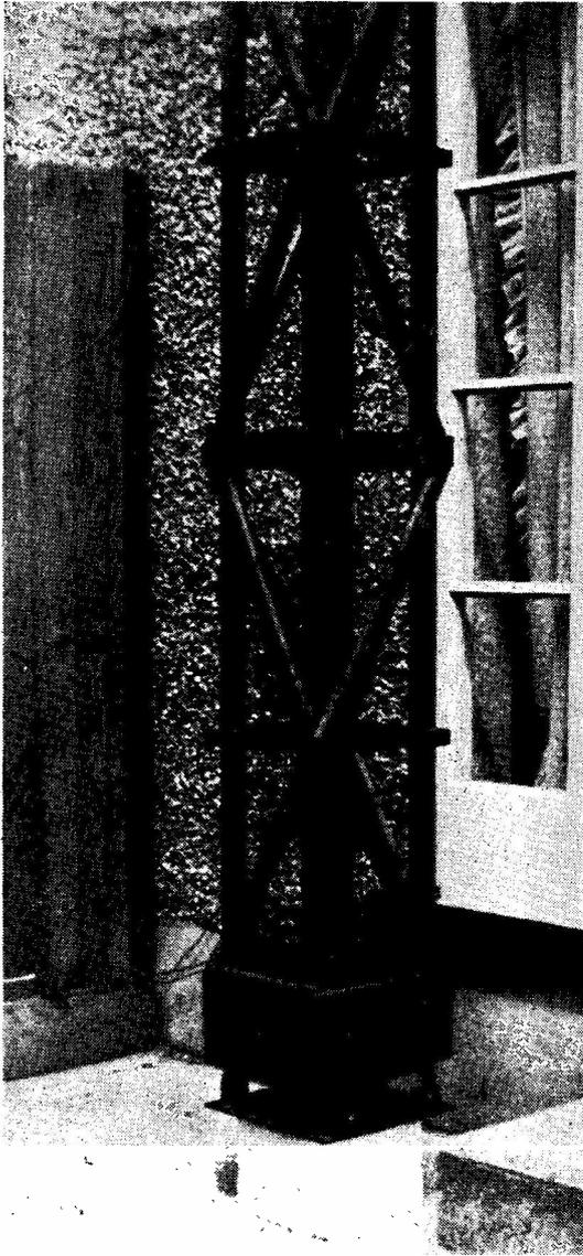
Photograph C. Showing the base assembly, consisting of a steel plate on a concrete block. By removing the two rear bolts and loosening the front pair, the tower can be lowered with the foot pivoted about these bolts.
