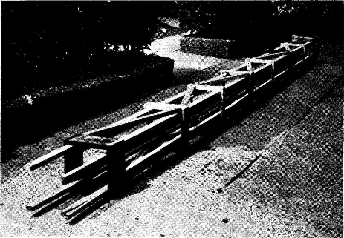
Photograph A. Showing how the near end is made to slide into the next box section. The essential feature of this design is that the tower can be elevated to its full height after having been raised to the vertical.
