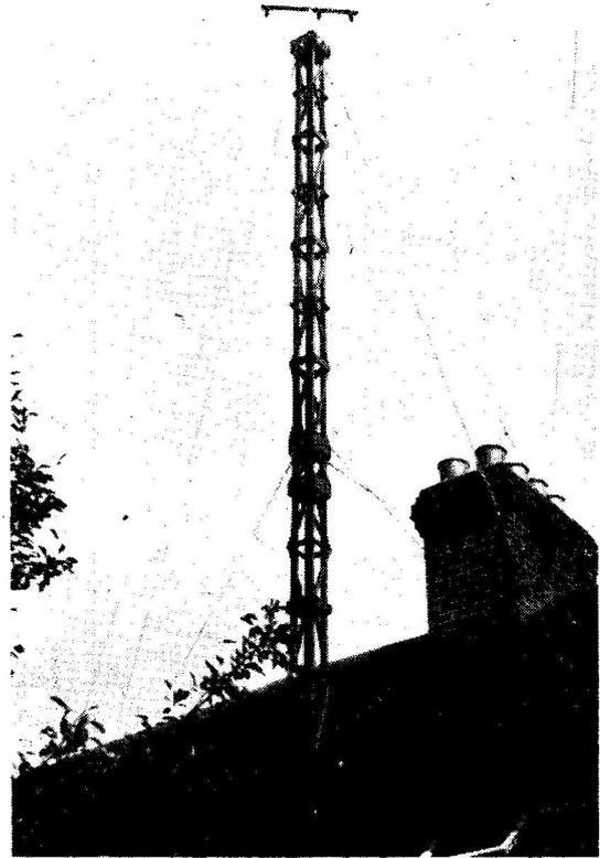
Photograph D. An impression of the whole assembly, as constructed and described by G3SM in his article, showing the guy-wire layout.
