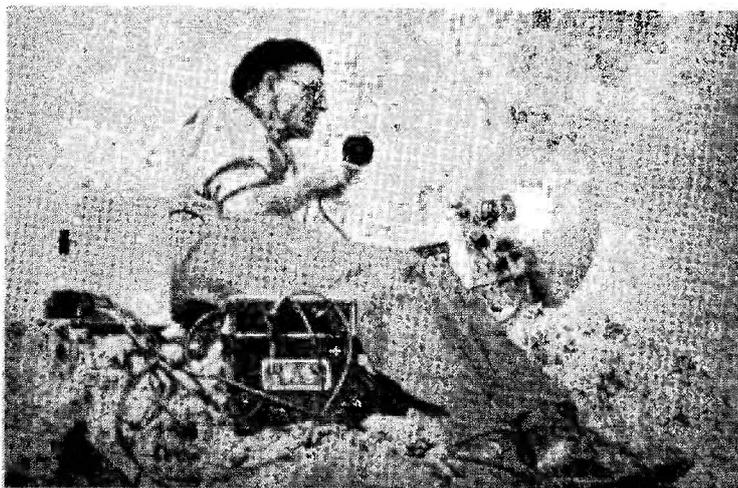
Other end of the 1250 mc 100-mile QSO. G3QC/P on Higher Fair Snape, near Lancaster on July 26, when at 1225 BST contact was effected with G8DD/P near Ludlow. Equipment at both stations consisted of a CV90 in a cavity oscillator, a super-regenerative receiver, and paraboloid beams. Each station had three helpers. It was in October, 1950, that the same two operators worked over a 75-mile path in the 1250 mc band, setting up a new record.
