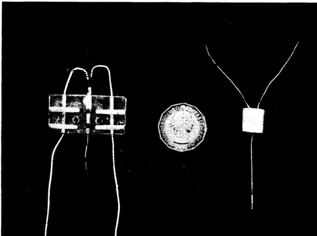
At left, the home-made transistor, as constructed by G3HMO. The crystal itself is just above the centre-line through the perspex block, which is used simply as a support for the germanium triode and its electrodes. At right is a commercial transistor, the G.E.C. GET-1 germanium triode. The 3d. piece is for size comparison.
