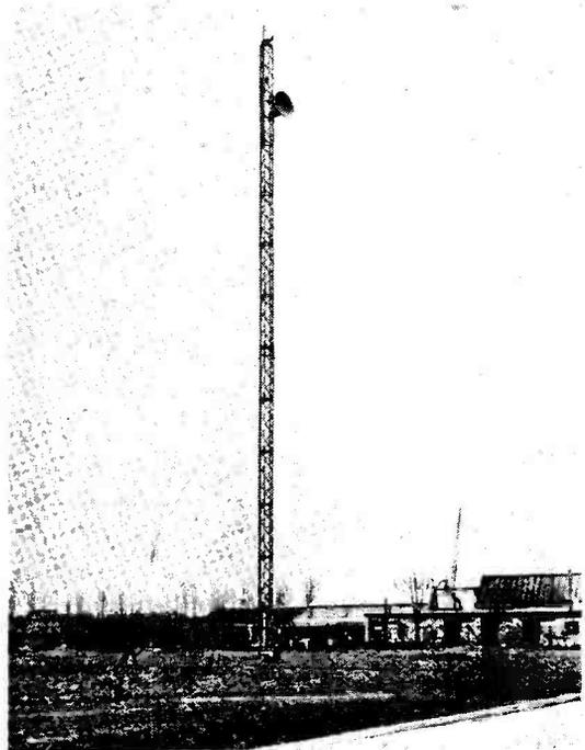
This is a B.I. Callender's Cable photograph of an aluminium mast built by the Northern Aluminium Co., Ltd. of Banbury, Oxon., for experimental HF/VHF work and the surveying of VHF paths. A mast of this type can be taken up to 200 feet.
