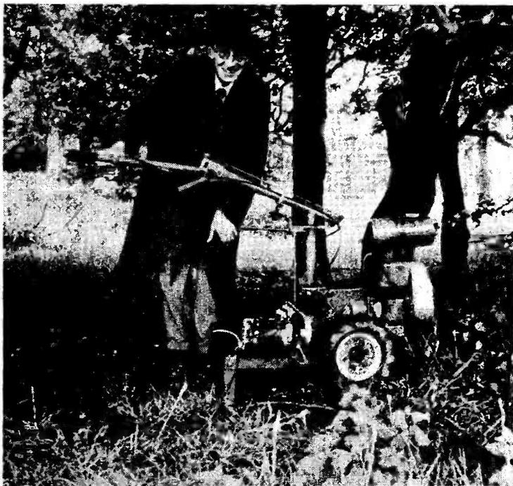
When the G3GVF party was out portable on Hannington Hill on June 6 last, they had a generator power supply driven by the engine of a hand-cultivator. Here is old timer G6OU setting the throttle.
