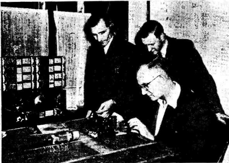
G2AUA demonstrating his transistor transmitter, running about 85 milliwatts input, at Wellingborough recently. The valve in the foreground (which has nothing to do with it!) is an 813, which can handle 250 watts quite comfortably. G2AUA is one of those experimenting with home-made transistors.
