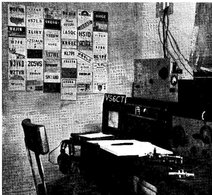
VS6CT is located at Little Sai Wan, Hong-Kong, and is actually the station of the local R.A.F. Amateur Radio Club, formed in November 1953. Original members were VS6DE (ex-G3HRY), VE5BQ, G3KGM and G3KLP (when serving in VS6). The receiver is an AR88 and operation is on 40 and 20 metres running 25 watts in a VFO/BA/FD/PA layout, with a selection of aerials.
