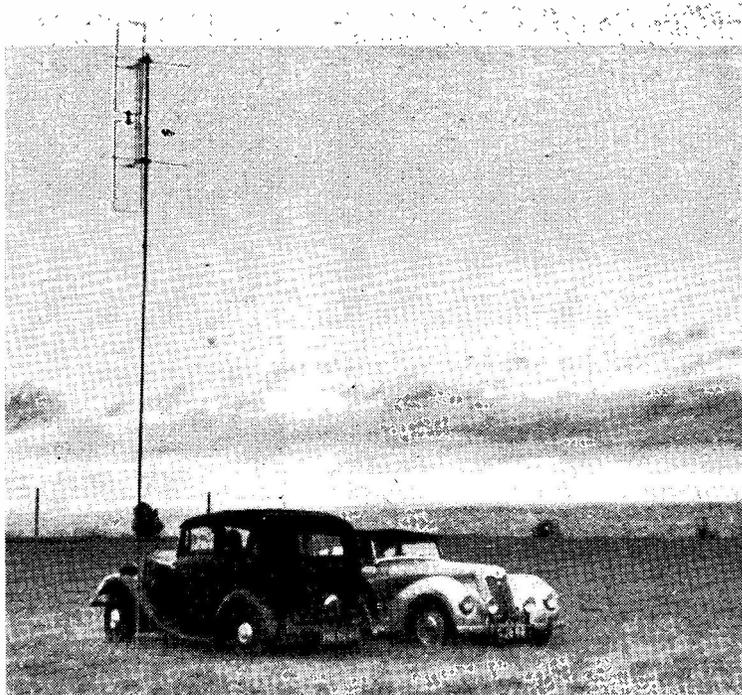
G8PX/P on Two Metres, with a portable Skeleton Slot assembly which put out a very potent signal from a site near Oxford on the field day of May 1st.
