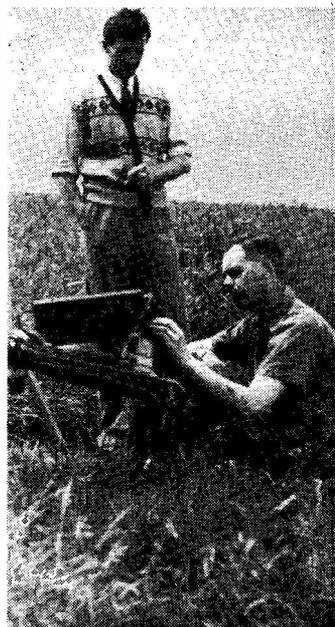
The G2CVD/P equipment for two metres consists of a 5w. transmitter using a 5763 and a double-superhet receiver, all built into an ASB4 case. Here we see G3BA operating and G2CVD looking on. With G3EJO, who took this photograph, G2CVD will be /P in Devon in late September, investigating various sites for portable work. Your A.J.D. suggests Dunkery Beacon, Hartland Point and the high ground near Torrington as likely spots that worked well in the old 5-metre days!
