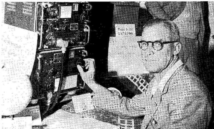
If you heard or worked ZS5DHE during July 8-16, it was the station of the Durban Radio and TV Society, at the Durban Crafts Fair. Transmitters were in operation on 3.5 and 7 mc, and here we see ZS5BF with the 80-metre equipment. In spite of the very high local noise level, usual on these occasions, a large number of contacts were made by the nine ZS's who manned the station.
