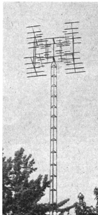
How they do it in Canada. VE3DIR, Toronto, has an all-VHF-band beam assembly, consisting of a 5/5 by 5/5 for each of the bands 144, 220 and 430 mc. Bays and arrays are at wavelength spacing and the whole erection, on a home-built mast about 40 ft. high, is rotated about the point of balance.
