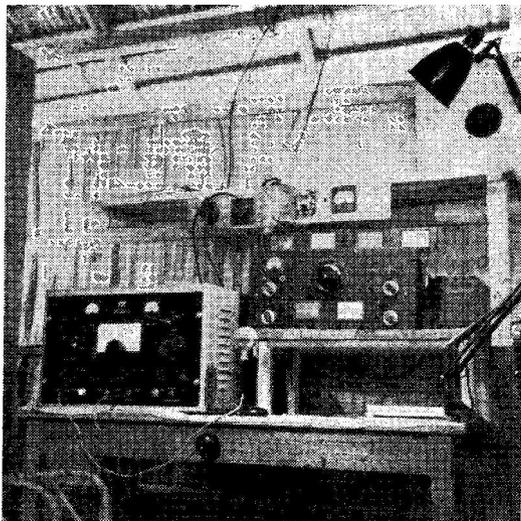
Station of VS5CT, in Brunei, British North Borneo. The transmitter was a modified Panda and the receiver an HRO. With the set-up as pictured here, some 536 contacts were made in 60 countries in two months on the site.
