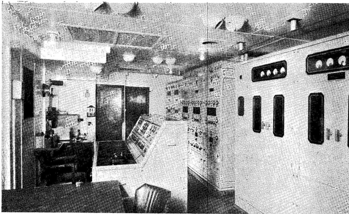
An impression of the remote-controlled transmitter equipment in the R.M.S. "Queen Elizabeth." The transmitters are normally unattended. In the far left-hand corner is the entirely separate battery-operated installation for emergency operation on the 600-metre band. The whole of the radio apparatus in the "Queen Elizabeth" and her famous sister the "Queen Mary" was supplied and installed by The International Marine Radio Company, Ltd.
