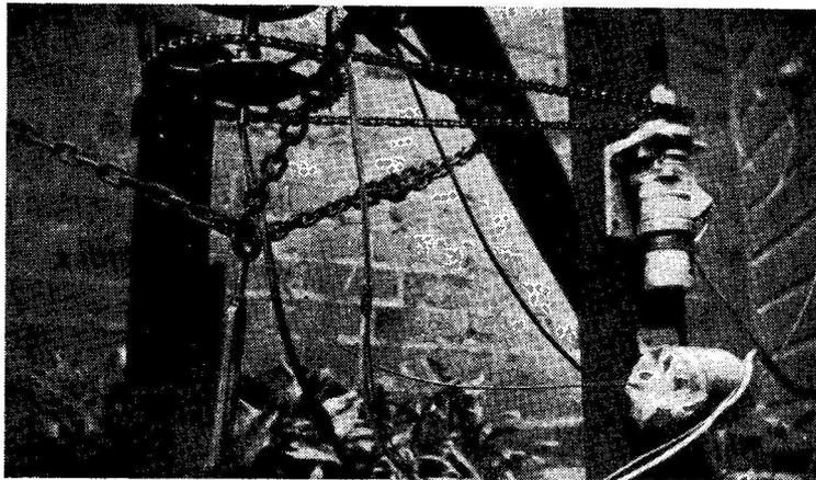
Base mounting and beam rotation gear at G3GSO, Derby. The head is a slot-fed 4-over-4 which, compared with the old 4-ele flat top, is giving very good results on two metres.
