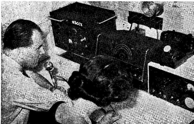
GC3CX is at Littlehampton, Sussex, the transmitter running a 6146 in the PA at 35w. input, modulated plate-and-screen by a pair of 6L6's; all bands 10 to 80 metres are used, with three aerials, and the gear is fully TVI-proof. Operation is mainly on phone. As we see from this photograph, the office work is handled by the XYL.
