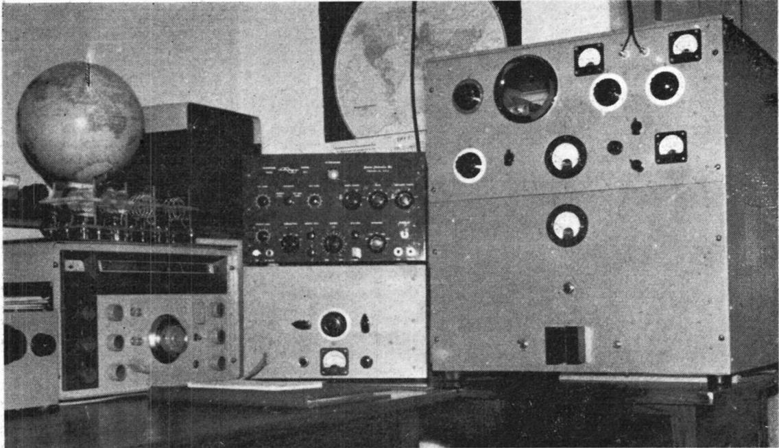
This is another view of the station of ZE5JJ, Salisbury, Southern Rhodesia, featured in the heading to "DX Commentary" in the April issue. Operating on SSB, the transmitter side consists of a home-built VFO into a commercial SSB exciter unit, driving an 805 as PA in the Class-B zero-bias linear arrangement. The receiver is a National NC300, and the station is fully voice-controlled. The aerials at ZE5JJ include a 3-element beam for 20 metres, with dipoles for the 15- and 10-metre bands.
