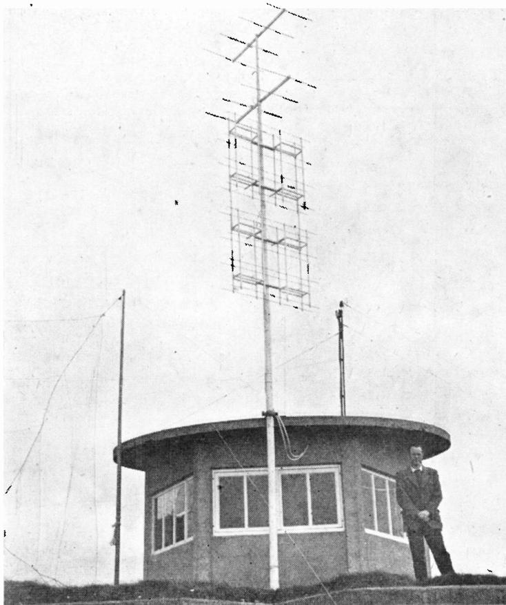
One of the best-known Europeans on two metres is F8MX, who operates /A during the summer from this fine site at St. Valery-en-Caux, overlooking the Channel. The two-metre beam is a 4-over-4, and the 70-centimetre array a 64-element stack; he also has a 70 cm horn, to the left, but not visible here. F8MX/F9CQ are brothers and have been very successful on VHF; both were present at the recent London VHF convention.
