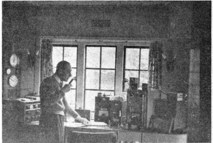
Having moved, G3HCU is now set up at his new QTH at Peaslake, Surrey. Visible are the beam direction indicator and 24-hour clock, and the AR88, at left, next the Top Band and two-metre gear, then the LG-300 transmitter and BC-221 frequency metre. The aerial system includes beams for 10, 15 and 20 metres (under construction) a G8KW multi-band, and a 256 ft. wire for 160 metres. All the equipment is relay-controlled by switches on the desk panels.
