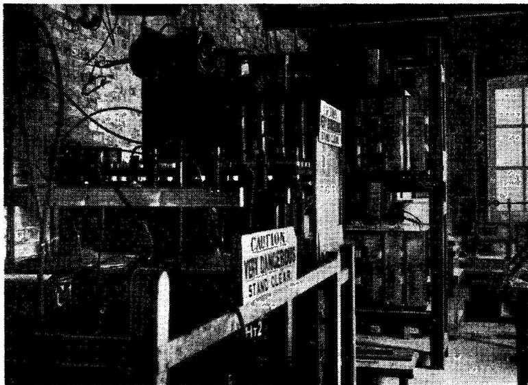
Marconi's spark transmitter at Poldhu, Cornwall, in December 1901, operating on a wavelength of "1200 to 1800 metres, not known exactly." The voltage across the spark-gap (right background) was 20,000v. and the transmitter was rated at 25 kW. It was this transmitter that put the first signal across the Atlantic, on December 12, 1901.
