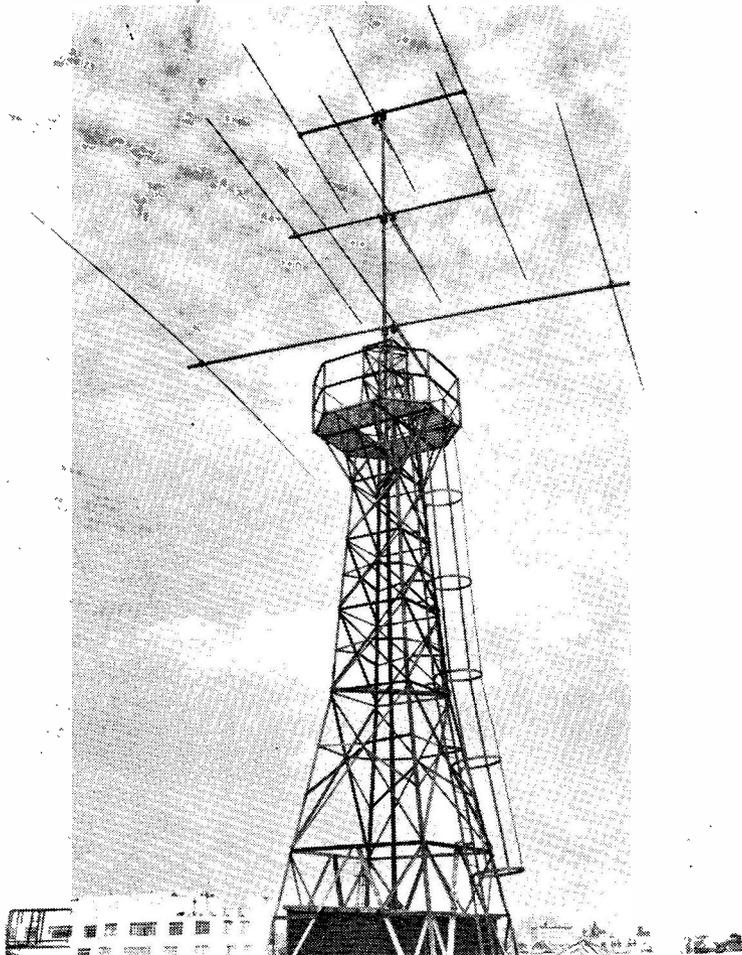
Three-band transmitting array for GB2SM, Science Museum, South Kensington, London, S.W.7. The tower, supplied by British Insulated Callender's Cables, Ltd., is 48 ft. over roof level, putting the 10-metre section of the array about 160 feet above the pavement. The other two sections are for 15 and 20 metres respectively. Having a separate, properly matched and fed, beam for each band has given GB2SM a much-improved DX potential.
