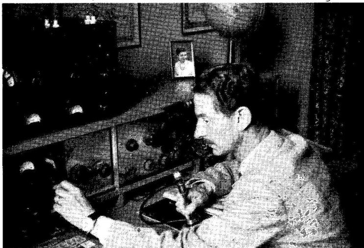
Station of 111T, Florence. This photograph was taken by SWL Paterson, G-L018, on a recent visit. He reports that 111T runs 150 watts in the transmitter and has a 12-valve communications receiver, all home-constructed. Aerials are a 20-metre Zepp, a dipole for 15 metres, and two-element rotary beams for 10 and 20 metres.
