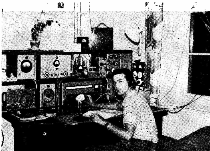
Station of DL6DZ, Caustrop Rauxel, in the Ruhr, who has been licensed about three years. He runs a Geloso VFO-807 PA transmitter, at 50w., for the HF bands and is also equipped for two metres. The receiver is the German RX-57, a modern communications type designed to D.A.R.C. specification. On the 10-15-20 metre bands, DL6DZ has two dipoles at right angles for each, also a tuned doublet fed with 600-ohm line. His main interest is phone and CW working on the HF bands, helped by a good knowledge of English. Though DL6DZ QSL's 100%, for all first contacts, and is now working for his WBC, he complains that far too many U.K. operators fail to reciprocate with a card. So if you owe him one . . .
